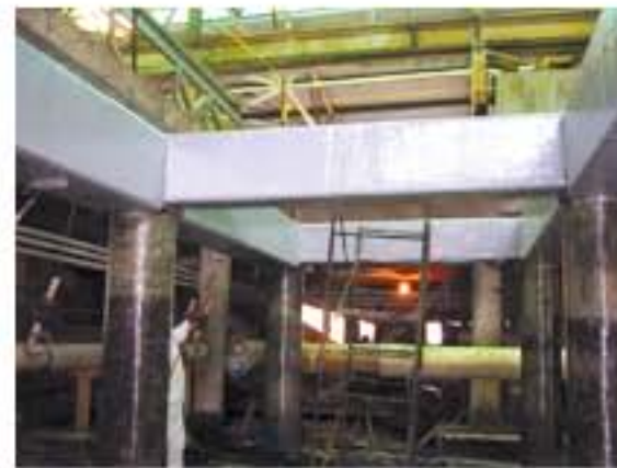
The CarbonSeal carbon fiber is lightweight, flexible and conforms to the substrate for easy installation
