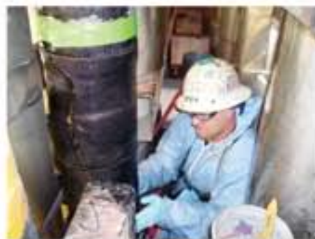
CarbonSeal Systems are designed for multiple pipe configurations including tees, elbows, straight runs, 90's, and blind flanges
