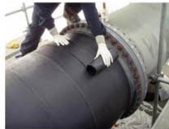
The CarbonSeal carbon fiber is lightweight, flexible and conforms to the pipe for easy installation
