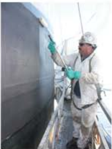
The CarbonSeal Steel Tank Repair System can be applied to the inside surface of a steel tank and the outside surface
