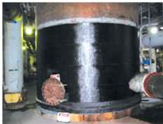
The CarbonSeal Steel Tank Repair System is resistant to corrosion and aggressive chemicals, so no future maintenance is needed on the repair
